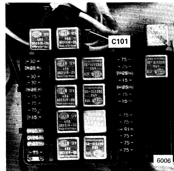
Figure 1 - Top Of Left Front Wheel Well
