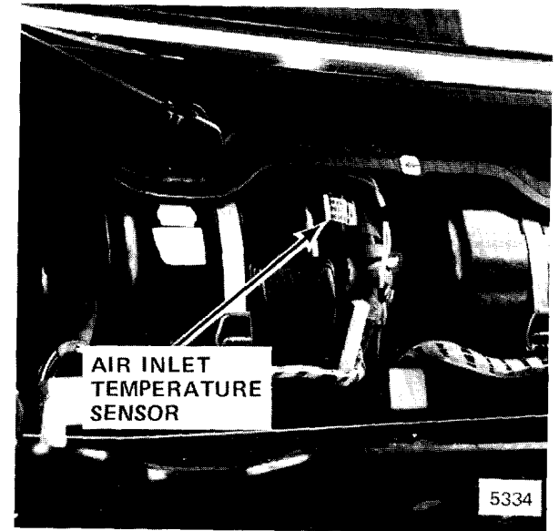
Figure 5 - Under Center Of Fresh Air Intake Cowl
