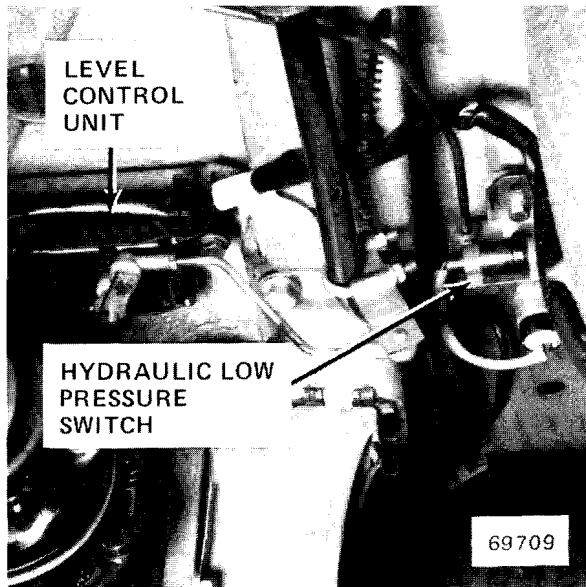
Figure 2 - Underside of Car, in Front of Fuel Tank
